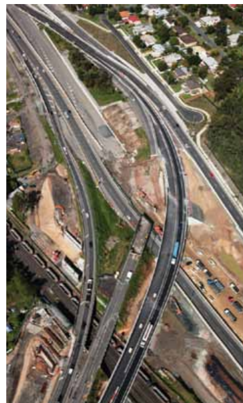
Part of the 'D2G' Ipswich Motorway upgrade, facing East.
